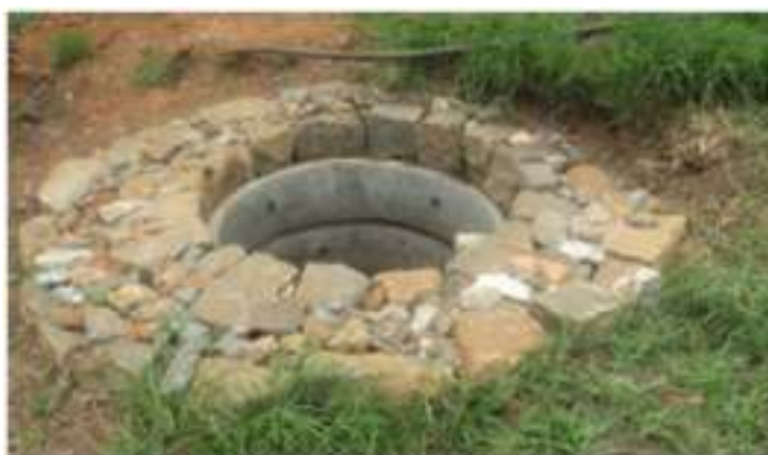
Soak pit provided for waste water from the factory
